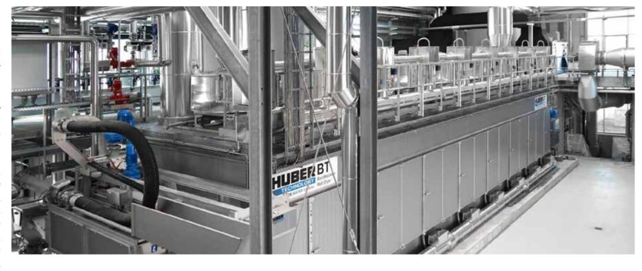
dry all the digested sludge post dewatering. A HUBER BT12 Belt Dryer was selected for the process.
